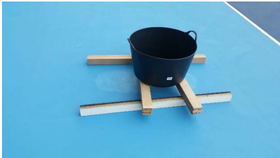
Protection of the surface where further leaks fall while allowing proper ventilation and drying where other leaks had fallen.
